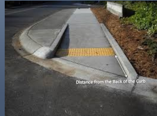
New ADA Compliant Ramp
