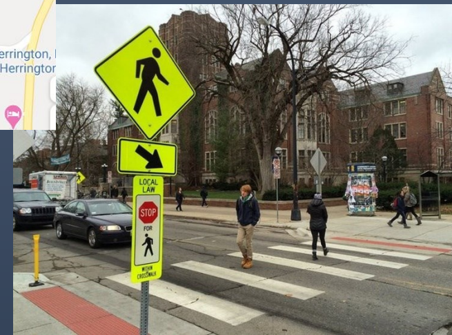
New Crosswalk/ADA Ramp
